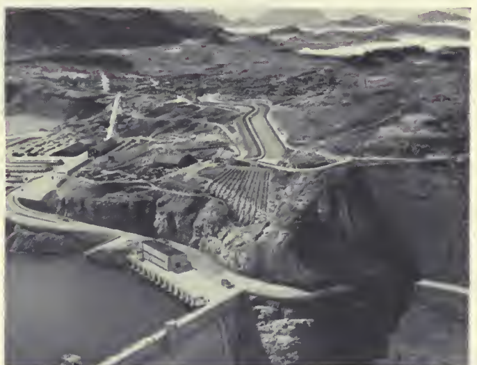
Coulee in the background, thereby reentering its ice-age channel, and forming an active storage reservoir for 1,202,000 acre-feet of water. Two earthfill dams, 27 miles apart, will seal the coulee as a reservoir. The first two pumps will require almost 3 months to fill the reservoir to a depth that will push water over the sill of South Dam, thence into the Main Canal which feeds the irrigation project. Both photos by F. B. Pomeroy, Region 1 photographer; art work by Russ Ducette, also of Region 1.
